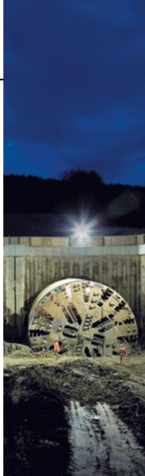
Katzenbergtunnel Parallel drive with two TBMs with EPB shields for the extension of the Karlsruhe–Basel motorway.
