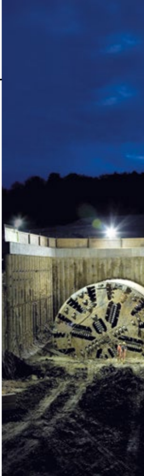
Katzenbergtunnel Parallel drive with two TBMs with EPB shields for the extension of the Karlsruhe–Basel motorway.
