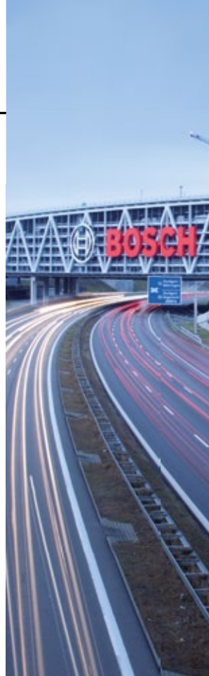
Car Park Neue Messe Stuttgart The Car Park Messe Stuttgart was constructed by using the cantilever construction method during ongoing traffic on BAB 8 motorway. The multi-storey building offers 4,000 parking positions and has a width of 100 m. The building was executed in 30 months construction time.
